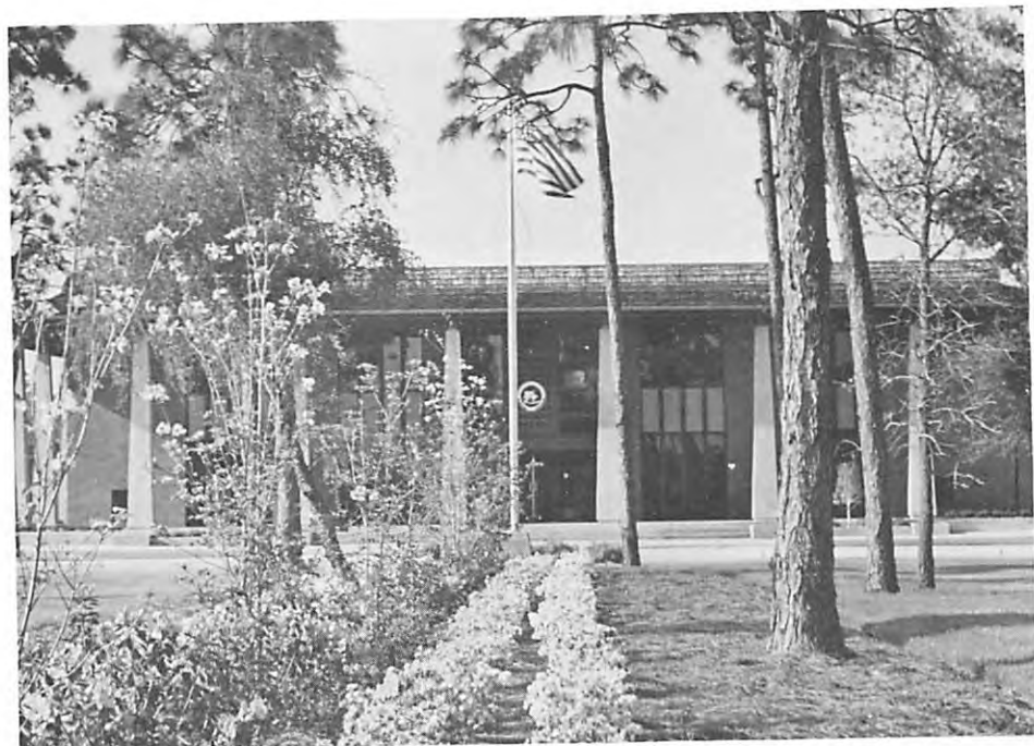
OWJC Administration Building
