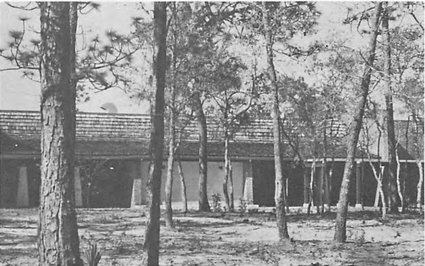
OWJC Heavy Shops Industrial-Technical Building.
